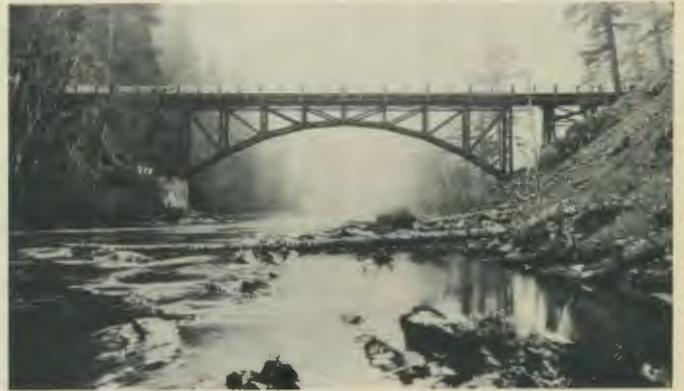
Structural engineers specify Douglas fir timbers, graded for strength and available in long lengths. This Teco ring-connected, arch-type bridge of treated Douglas fir has a 135-foot span.
