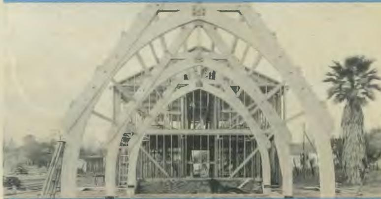
Glued-laminated Douglas fir can be engineered for strength and designed for beauty. As the framework of this Southern California church indicates, it can be fabricated into a wide variety of sizes and shapes.
