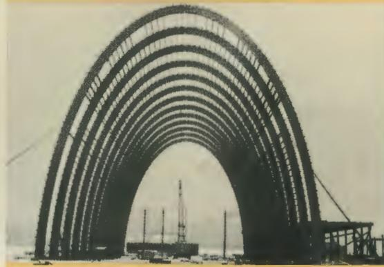
Wood engineering produces spectacular results. The Radar Test Laboratory, Dayton, Ohio, used glued-laminated Douglas fir lumber for stability and permanence.
