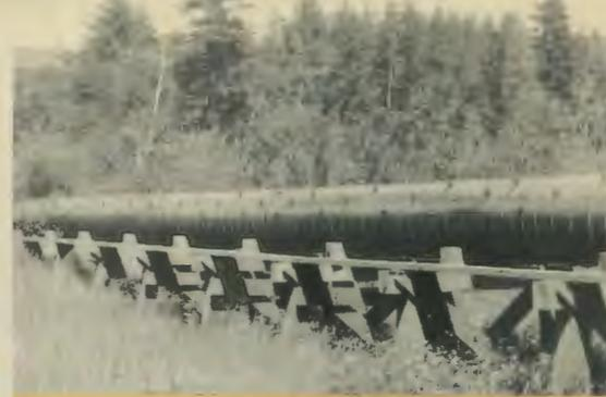
If it's a woodstave pipe it may be Douglas fir, treated or untreated, or Western red cedar. Both are widely used for flumes, water and septic tanks—wherever strength and durability are required.
