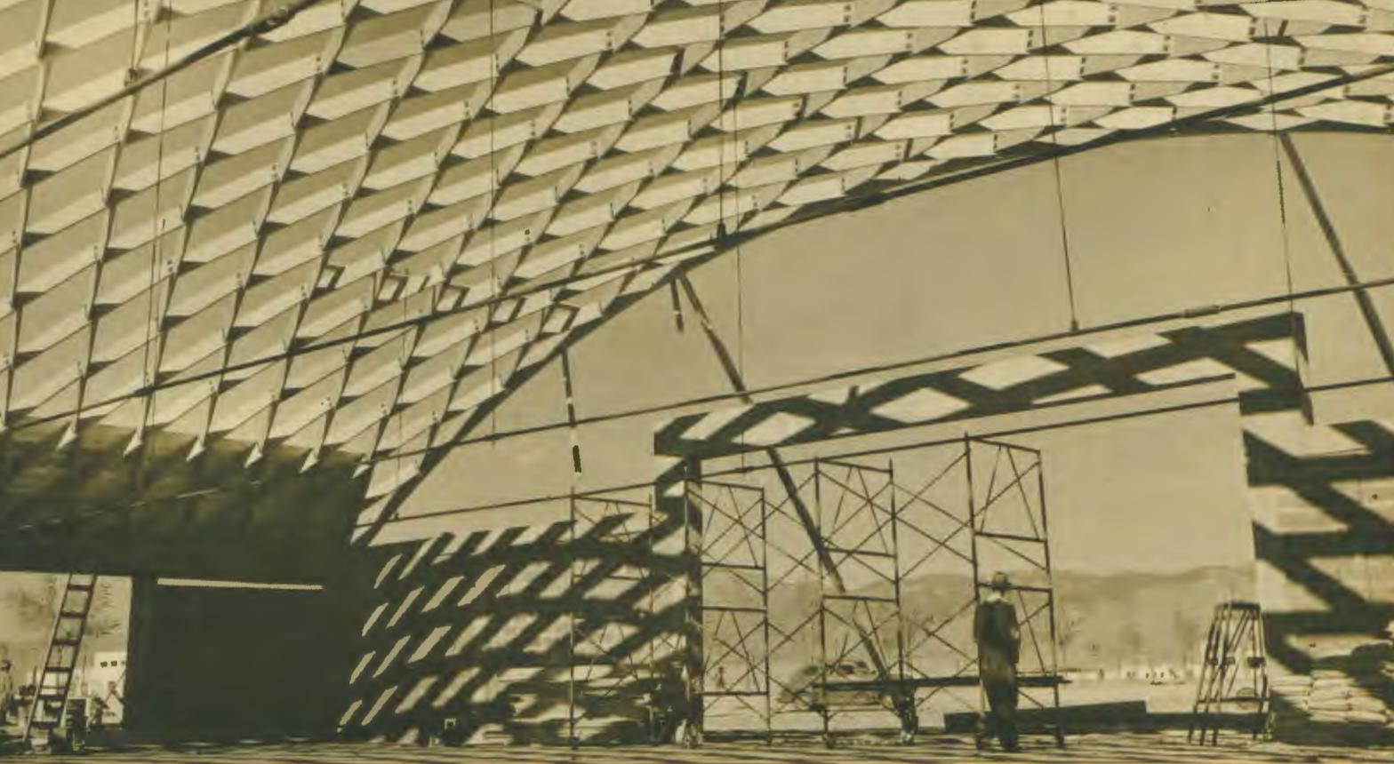
**Industrial innovations are steadily expanding the uses for West Coast Woods.** The eye is caught by streamlined examples of timber engineering such as this Lamella roof, one of several types of roof construction using Douglas fir. Wood is economical and long spans are possible.
