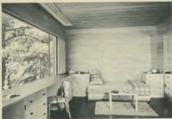
Striking and graceful effects are obtained when wood is coupled with the simplicity of modern design. This attractive study-dressing room, designed by Klaus Pfeffer, is paneled in vertical grain Douglas fir.
